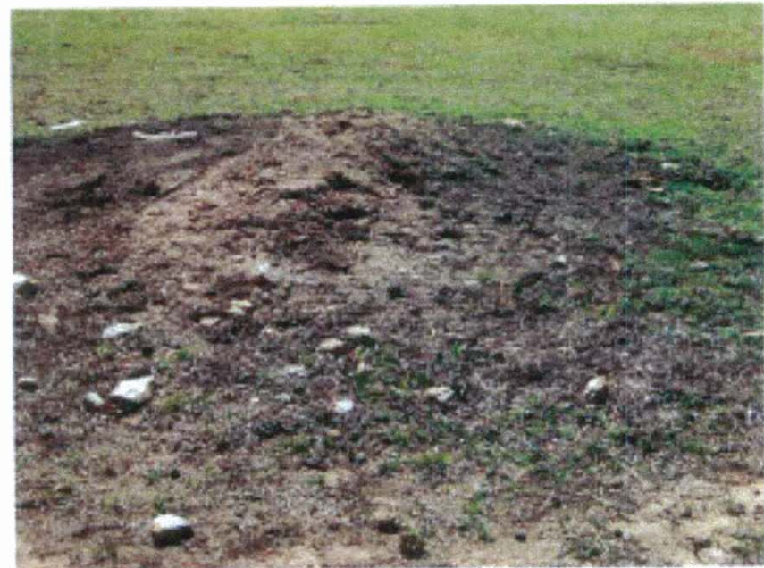
Grass cover in poor condition and large areas have been eroded.
