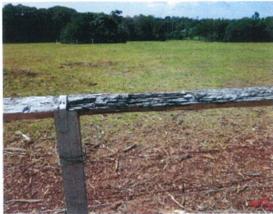
Fencing in very poor condition with evidence of white ant infestation.
