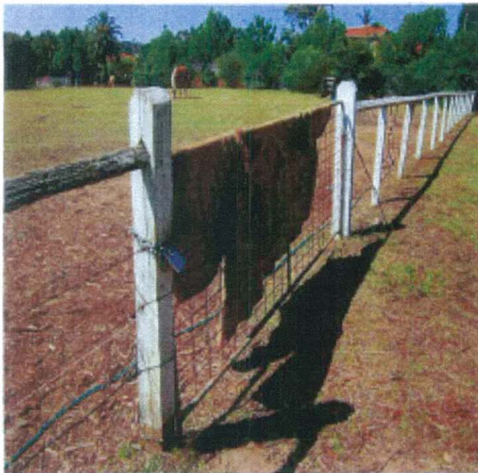
Fencing in very poor condition with evidence of white ant infestation.
